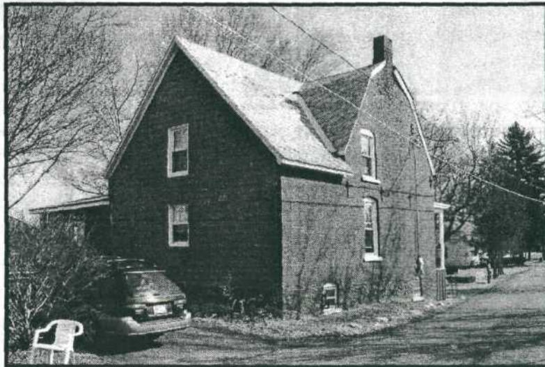
The Douw Fonda House Cohoes, Albany County, NY (back view)
